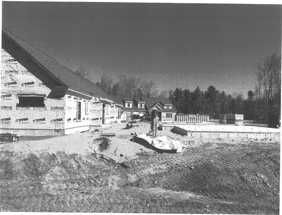
Looking towards Unit 5 (left framed) & Unit 8 (right foundation)
