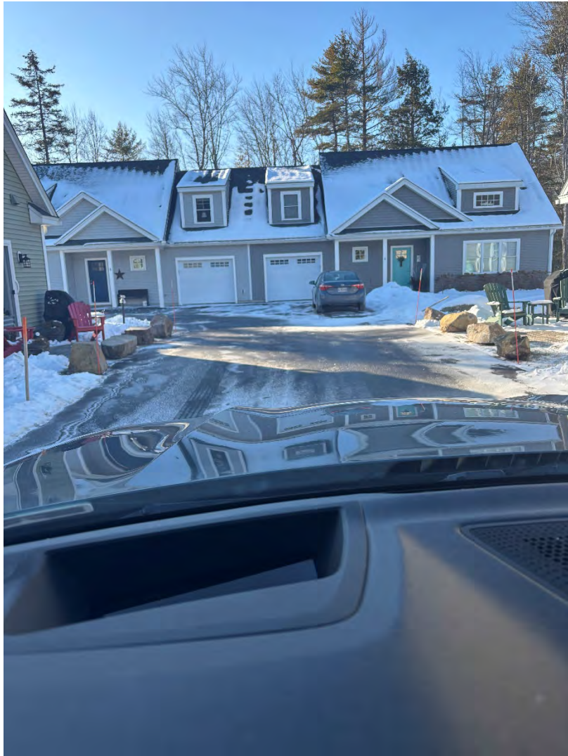
taken from: Izzys Lane, looking South down Izzys Lane view of Protective Boulders installed for Units #12 & #15
